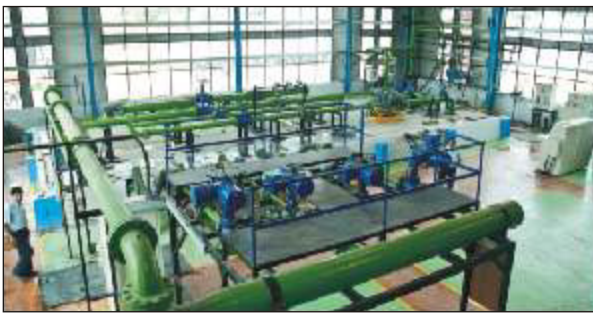
Type Testing Plant
