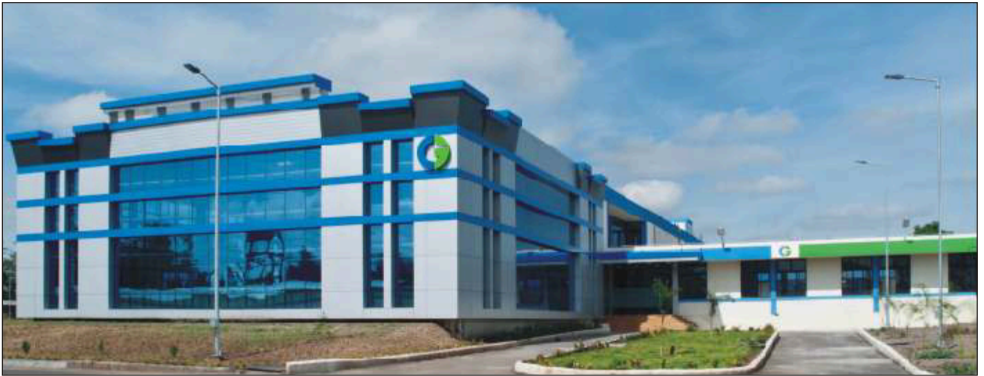
Manufacturing Plant, Ahmednagar
