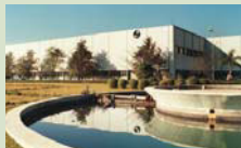
Switchgear Factory, Ahmednagar
