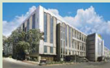
Powal Switchgear Factory, Mumbai
