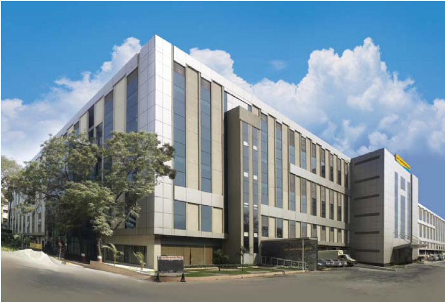
Switchgear Factory, Mumbai
