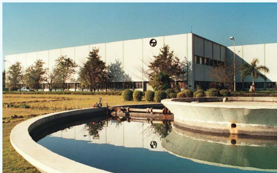
Switchgear Factory, Ahmednagar
